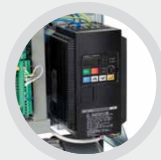
1.5KW power inverter integrated, easy to program permits to adjust precisely speeds, rump-up and rump-down times.
